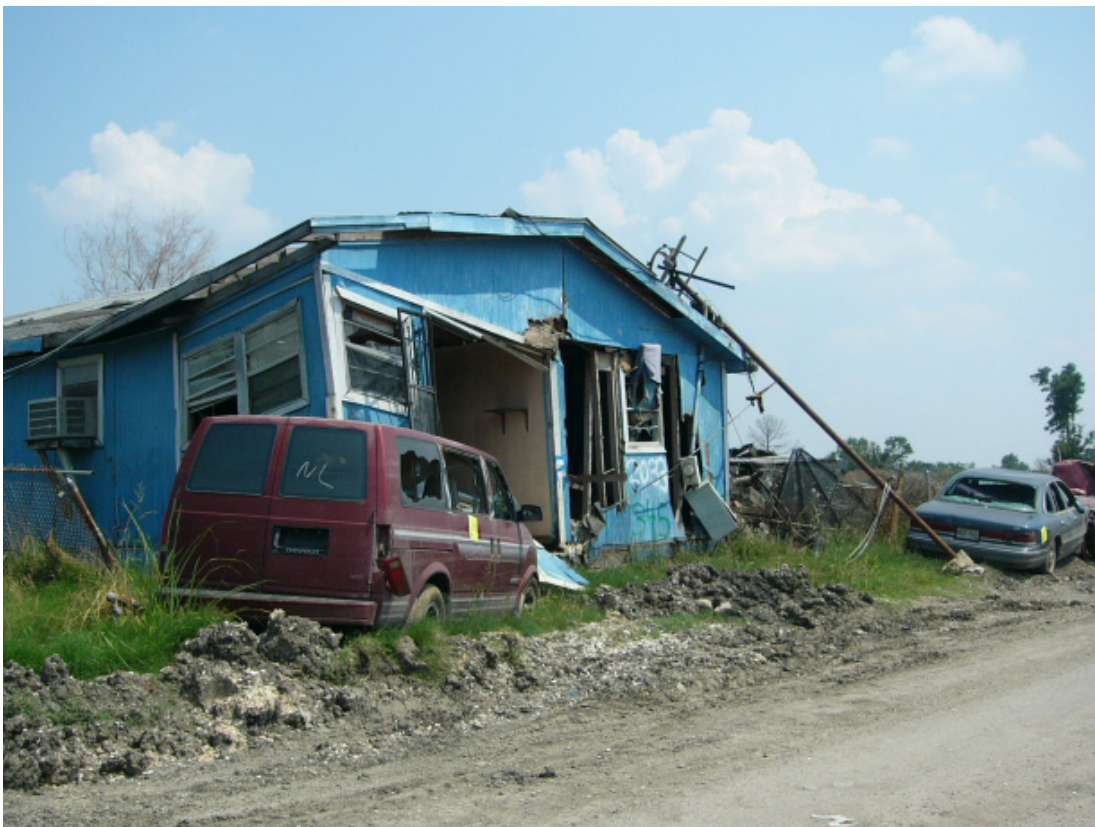
New Orleans 9th Ward, days after the floodwaters have receded, in a scene from Trouble the Water. Courtesy Elsewhere Films.
